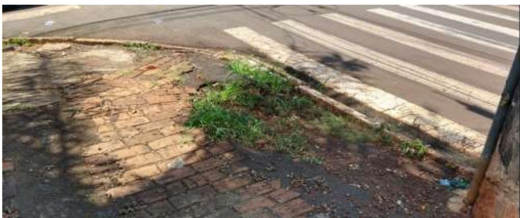
**Figura 12 – Calçada em extremo desnível e sem rampa – Av. Brasil**
