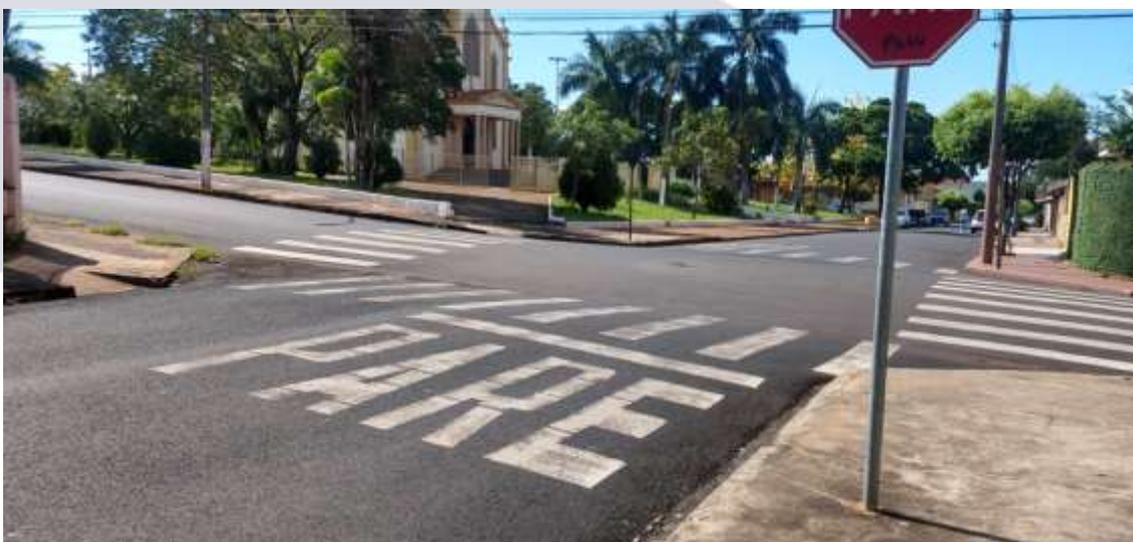
**Figura 80 – Travessia de pedestres sem acessibilidade**
