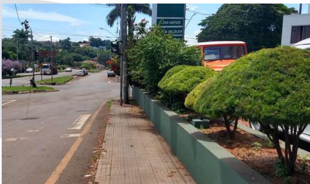
**Figura 11 – Faixa de pedestre sem acessibilidade – Av. Brasil**
